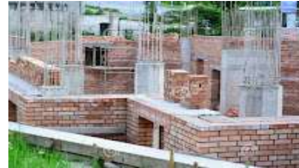
Case 2: Concrete frame construction with Hollow Clay Blocks - wall thickness 200 mm
